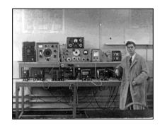
I was based at RAF Yatesbury, No2 Radio School, in Wiltshire just as the three V-Bombers came into service. I equipped two new labs each with six sets of fully working STR18's - here is one set on the lower bench (with a rather younger me - now 85) and associated test equipment above as was expected to be supplied to all Maintenance Units at operational airfields".
